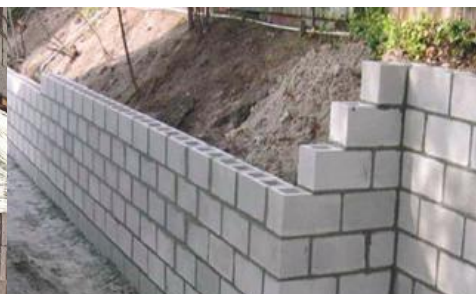
Increase Bricklaying Strength
