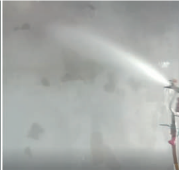
4. Spray water on skim coat surface to remove dust and to give a smooth and clean surface.
