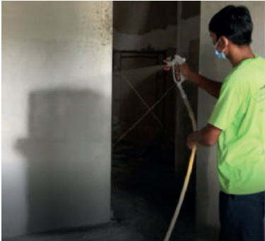
1. Spray TPS Grey Base Spray to surface.
