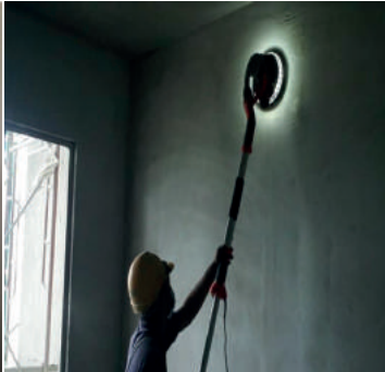
3. Polish with TPS Sander the next day to smoothen surface. Patch up surface when required.
