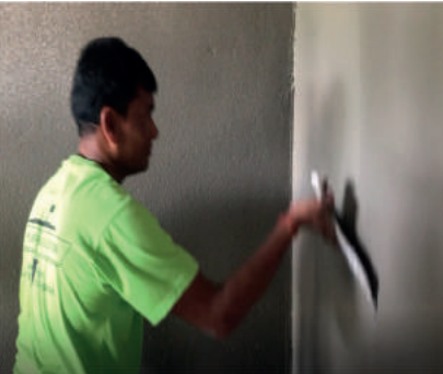
2. Trowel with wide filling knife or leveling knife to partially level the surface and reduce bubble hole on surface.
