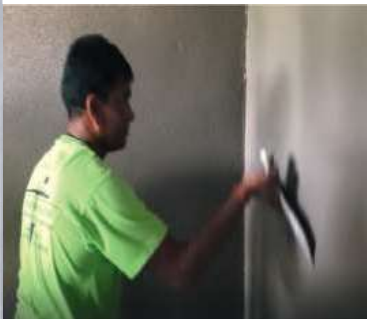
TPS Skim Coat can be trowel with wide filling knife
