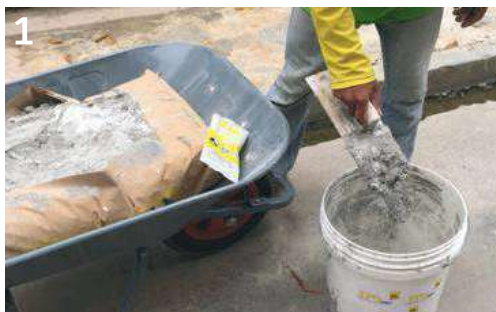
1 Mix TPS Yellow with cement in paint barrel. Mixing ratio based on application required.
