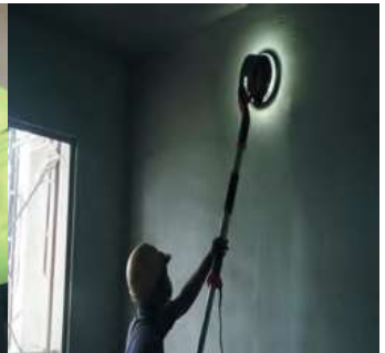
Can be polish with TPS Sander the next day to smoothen surface. Patch up surface when required.
