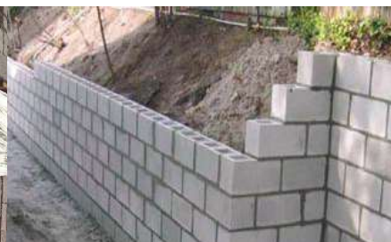
Increase Bricklaying Strength
